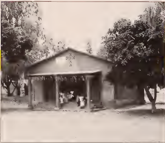
A sister church in Zaire recently erected through an African - PC(USA) partnership.
